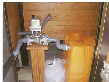
Urine separation in machine room
