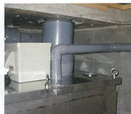
Processing tank and piping in the pit
